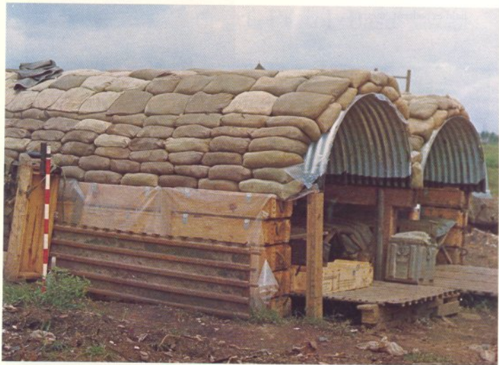
Personnel Bunkers Using Steel Culverts
